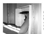
Position box and install a #10 screw (not included) in the upper left and right horizontal slots using the pilot holes. Adjust front edge of box 1" from the stud face and tighten screws. Install other two screws.
