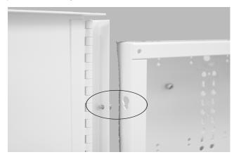
6. The box has 8 columns of repeated 2-hole patterns labeled A, B, D, E, F, H, J, & K (see diagram). In each 2-hole pattern one hole in slightly larger than the other. These are for plastic Circuit Board Glides (p/n ELK-SWG). The small hole fits a 6/32 type "F" mounting screw and the large hole is for the half-moon locator tab on the bottom of each glide.
