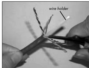
1. Carefully strip away approximately 30 mm of the cable jacket(s) (above left) to be connected to the Patch Panel, separating the wires into four pairs. Using a wire cutter, cut the wire holder (above right) flush with the cable jacket.
