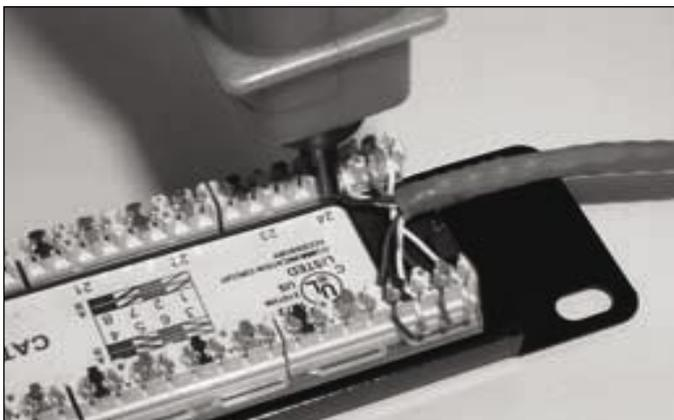
2. Follow the IDC color-code chart above to position the wires, then use a Krone punch-down tool to crimp and connect them.
