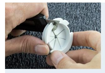
Use a utility knife when installing the grommet around preexisting cables. The grommet is designed to hold its shape after being split open.
