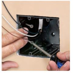
**3** Mount ONE-BOX directly to stud with shipped in place screws.
