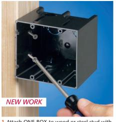
1 Attach ONE-BOX to wood or steel stud with captive installation screws. If the box is too far forward or back, simply back the screws out and reposition it.
