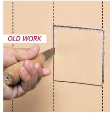
1 For old work, position ONE-BOX adjacent to stud. Use box as the template to cut hole.
