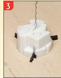
3 Add drop wire to loop. Attach to framing member above.
