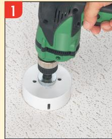
1 Cut hole in a ceiling grid with 4" hole saw. 4-1/2" for steel.
