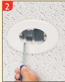
2 Install CAM-BOX™ kit. Rotate to desired position. Tighten mounting wing screws.
