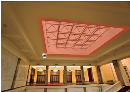
Skylight protection at Public facility / Warehouse
