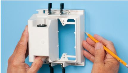
1 Use enclosure (without trim plate) as a template for opening. Cut hole.
