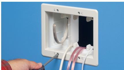
3 Tighten mounting wing screws to pull the box securely against the wall.
