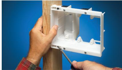
1 Attach box to stud using #6 screws. Use tabs on box for proper positioning of box depth.
