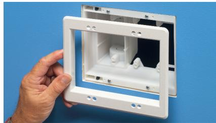
3 Attach paintable trim plate with screws provided. See below, left for reference.
