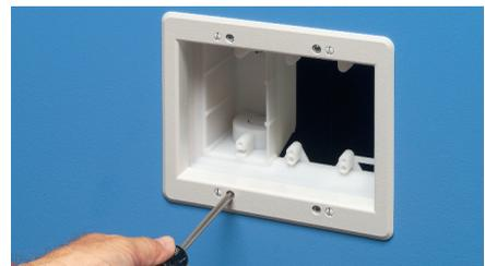
4 OPTION for new work: Tighten mounting wing screws to pull the box securely against the wall.
