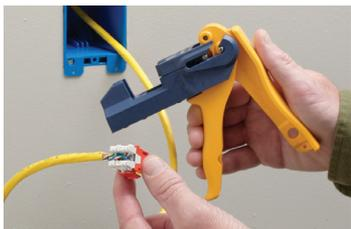
7. Release handle and remove jack from JackRapid tool. Visually verify proper termination.
