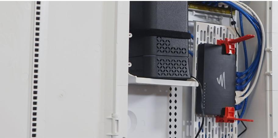
The latest in cable management and device mounting for 3<sup>rd</sup> party accessories within ON-Q enclosures. Mount devices and organize your enclosure with Forward Keyhole Post Clips and Small Device Mounting Clamps. Organize unsightly cables for a professional look and feel with the new Cable Channels. Explore the latest in ON-Q enclosure accessories below.
