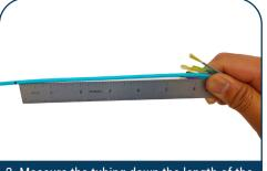
Measure the tubing down the length of the cable. Place a mark 6"/15 cm from the end of the tubing.
