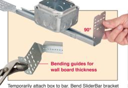
ends 90°, forward or back. Bend bracket ends again at the mark for desired wall board thickness.
