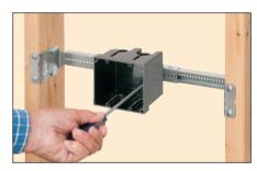
Install plastic or metal box(es) on SliderBar with #8 sheet metal screws.
