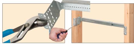
Bend bracket ends at 2-1/2" mark for use with 1/2" or 5/8" thick wall board. Ends can also be bent 90° or backwards (180°) as needed for inside mounting.
